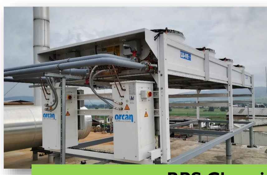
BPS Chornice Chladič eCooler 800 kW
